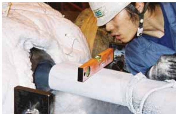
23. Commencing shrinkage fit (fitting time two seconds).
