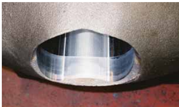
21. Interior of vertical connection before insertion.
