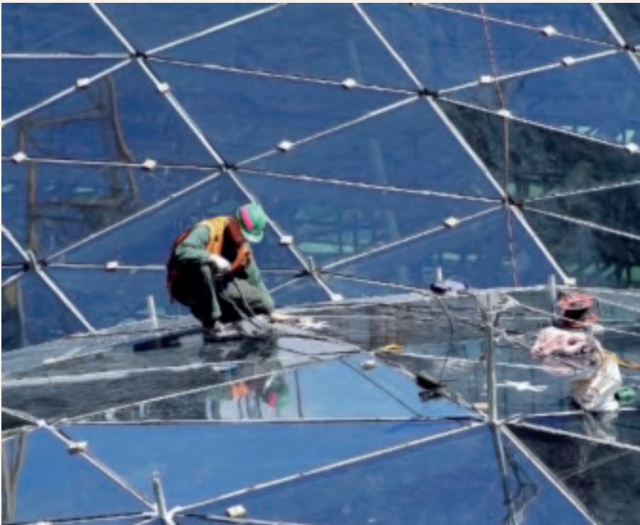
41. Glazing sealant installation.
