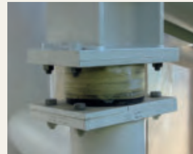
26. Elastomeric bearing at the drum bracket support.
