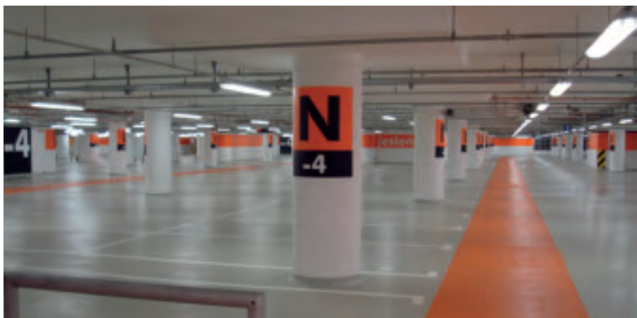
48. Basement level B4 car park, showing the drop heads to the columns.
