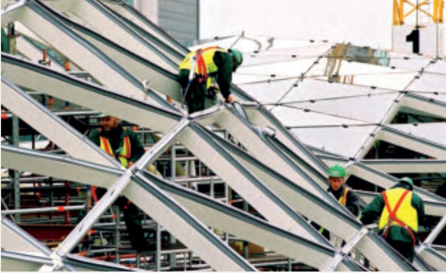
36. Glazing gasket installation.
