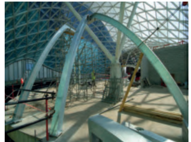
10. Steelwork under construction for the “Helmet”.
