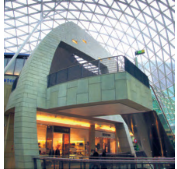
9. “Banana columns” for the “Bowl”, and cantilever support platform for escalators.
