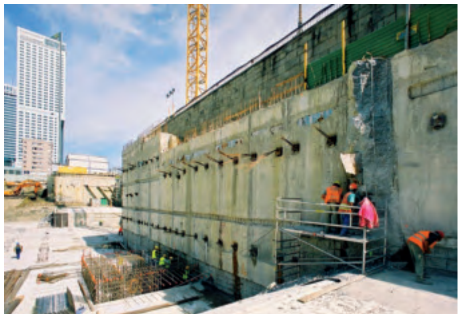
6. Diaphragm retaining wall with ground anchors, along the east edge of the site.
