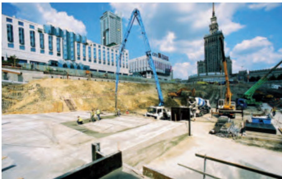
7. Raft foundation under construction at B4 level. On the left is the soil berm left in place to support the diaphragm wall along Złota Street, on the other side of which are the "City Center" shopping centre and the Holiday Inn Hotel.
