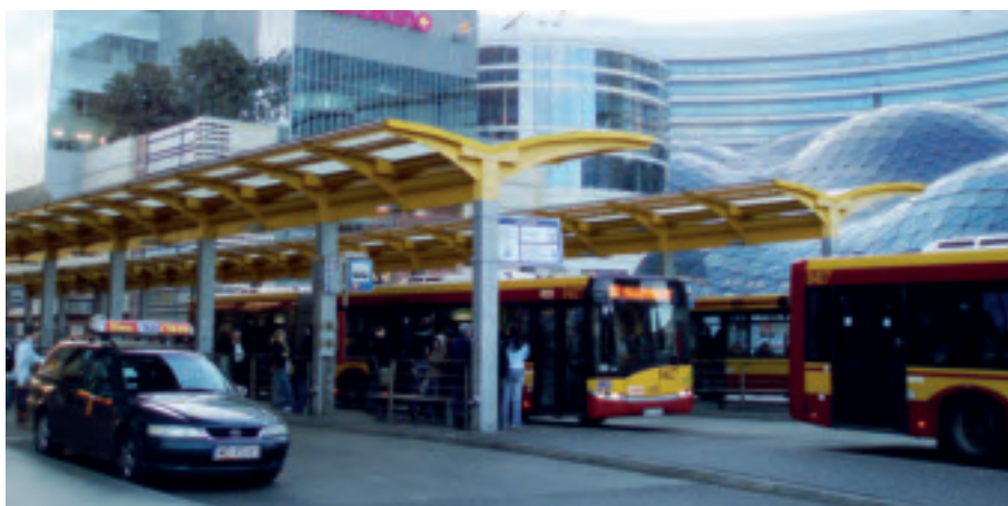
49. The new bus station.
