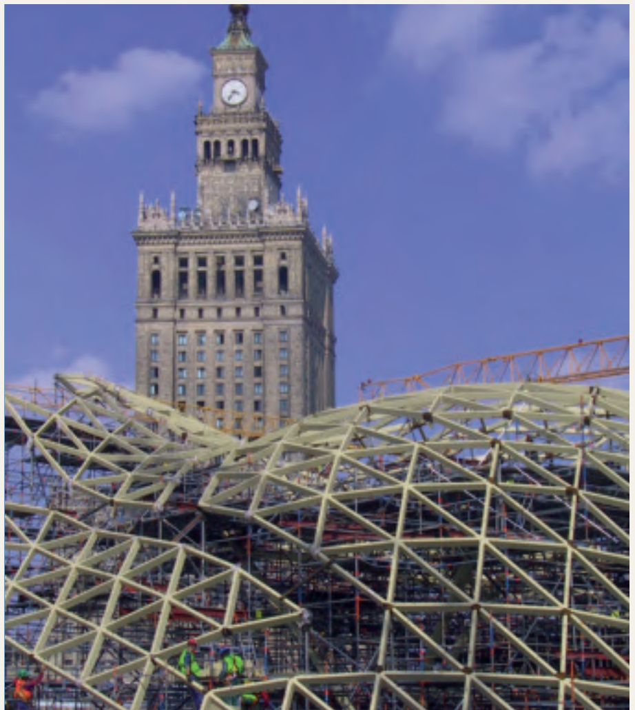
40. Erection of ladder frames.
