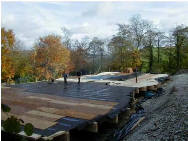
Figure A.38: Floor and beams are cut into shape. Image from [www.wealddown.co.uk](http://www.wealddown.co.uk)
