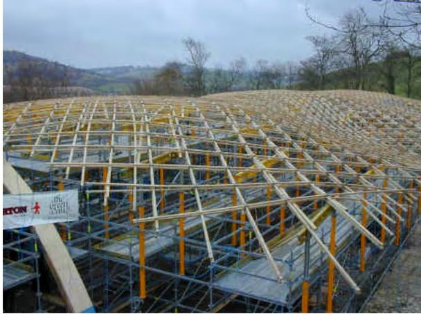
Figure A.44: Start of lowering. Image from [www.wealddown.co.uk](http://www.wealddown.co.uk)
