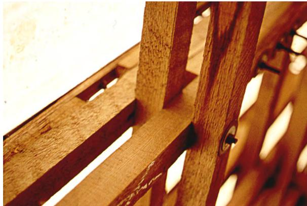
Figure A.17: Photo of a typical node joint. Image from [www.kunst.uni-stuttgart.de](http://www.kunst.uni-stuttgart.de)
