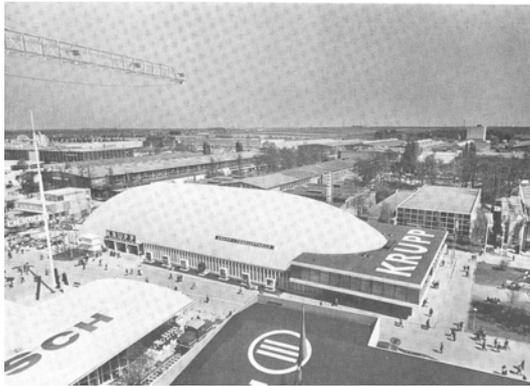
Figure 3.65: An exhibition hall by Krupp in Hannover, shape like a toroid (=part of a cylindrical ring).
