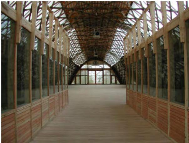
Figure A.33: The Weald & Downland grid shell. Image from [www.wealddown.co.uk](http://www.wealddown.co.uk)
