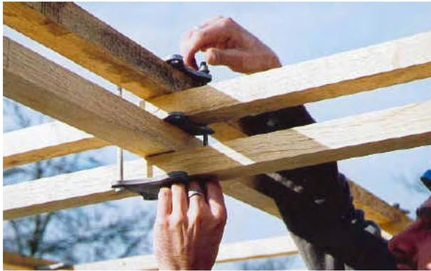
Figure A.37: Assembly of a typical node joint. Image from [www.wealddown.co.uk](http://www.wealddown.co.uk)
