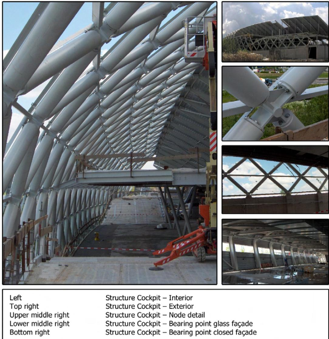
Figure A.85: Structure of the Hessing Cockpit
