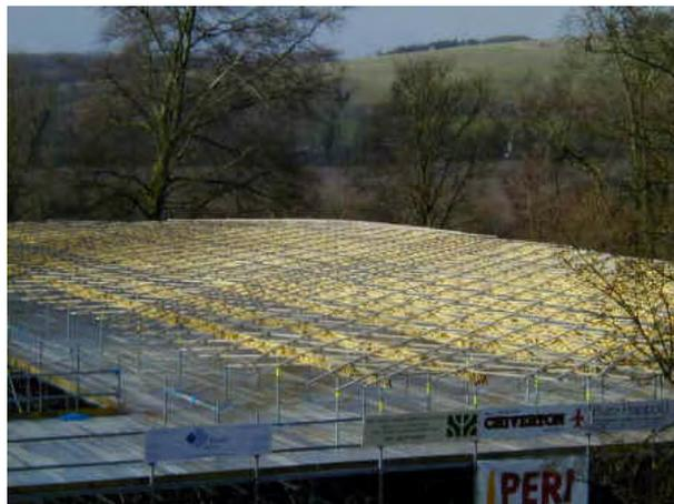
Figure A.43: Flat mat of laths. Image from [www.wealddown.co.uk](http://www.wealddown.co.uk)
