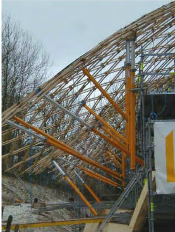
Figure A.46: Angled jacks. Image from [www.wealddown.co.uk](http://www.wealddown.co.uk)
