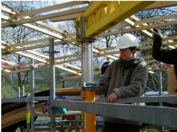
Figure A.45: Adjustable jack. Image from [www.wealddown.co.uk](http://www.wealddown.co.uk)
