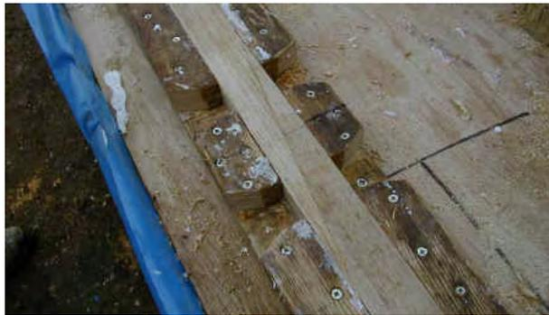
Figure A.36: Scarf joint. Image from [www.wealddown.co.uk](http://www.wealddown.co.uk)
