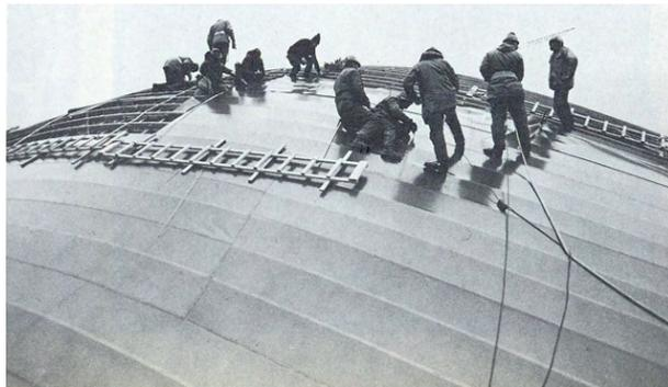
Figure A.25: Applying the roof skin. Image from Burkhardt et al. 1978
