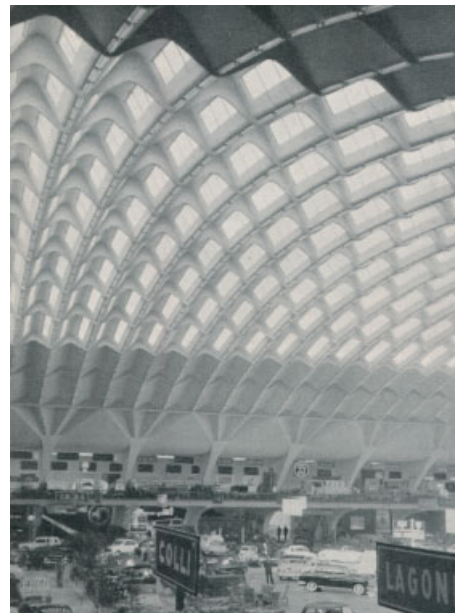
Pier Luigi Nervi, Exhibition Hall, Turin, Italy, 1949 The long span vaults were constructed using prefabricated ferro-cement panels to reduce on-site formwork.
