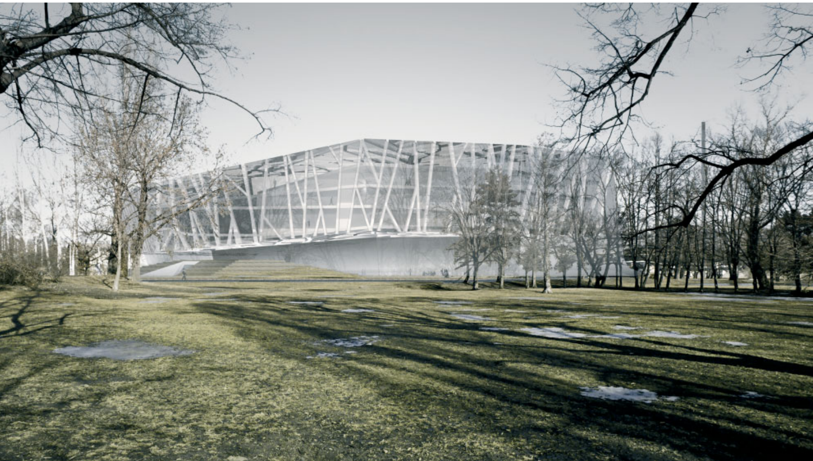
Exterior view of the library situated in Letenské Park showing the intricate branching structure derived through an integral computational form-generation process.
