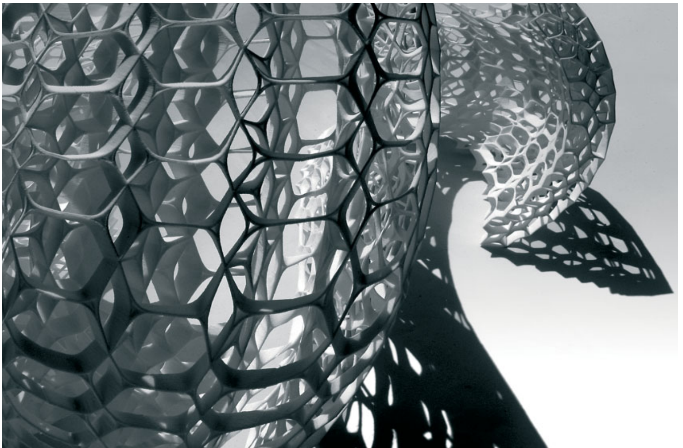
The Strip Morphologies screenwall, designed in 2005 by Daniel Coll I Capdevila of OCEAN, explores a multiple-layer, double-curved and variable-depth bent strip arrangement to modulate visual transparency and, luminous, thermal and acoustic performance, and enables layered spatial arrangements by means of a porous envelope.
