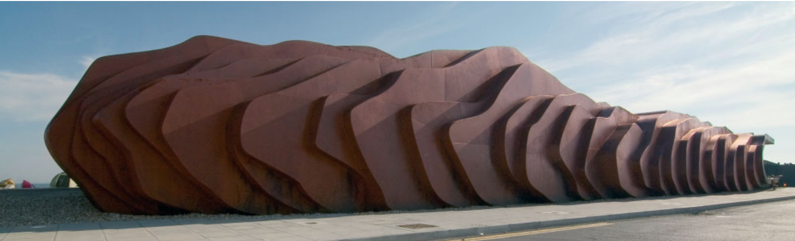
View of the building from the seafront car park. The mild steel has been finished with an oil-based coating, allowing for a rust-like patina without structural degradation.
