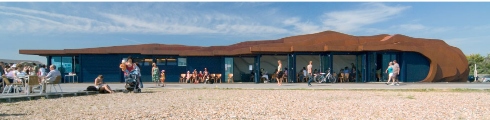
Heatherwick Studio and Adams Kara Taylor, East Beach Café, Littlehampton, West Sussex, 2007 The front of the café, seen from the beach. The left-hand end of the ribbons forms a canopy for the takeaway kiosk. Inside, white plasterwork follows the contours of the exterior shell.
