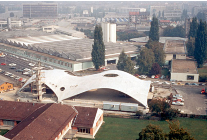
Heinz Isler, Factory for Sicli SA, Geneva, Switzerland, 1969 Isler's Sicli project demonstrates the unconventional geometries that can be found using fabric models.
