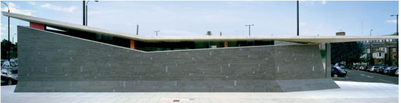
The long elevation of the building; from this angle, the purpose of the structure is unknowable.
