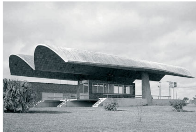
Eladio Dieste, Entrance canopy for Refrescos Del Norte, Uruguay, 1977 The floating roof form is constructed from a pair of freestanding barrel vaults, cantilevering from a single central row of columns. The vault is constructed from prestressed brick.
