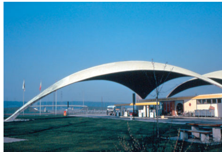
Heinz Isler, Service station, Deitingen Süd, Switzerland, 1968 The building consists of two symmetrical freeform concrete shells.
