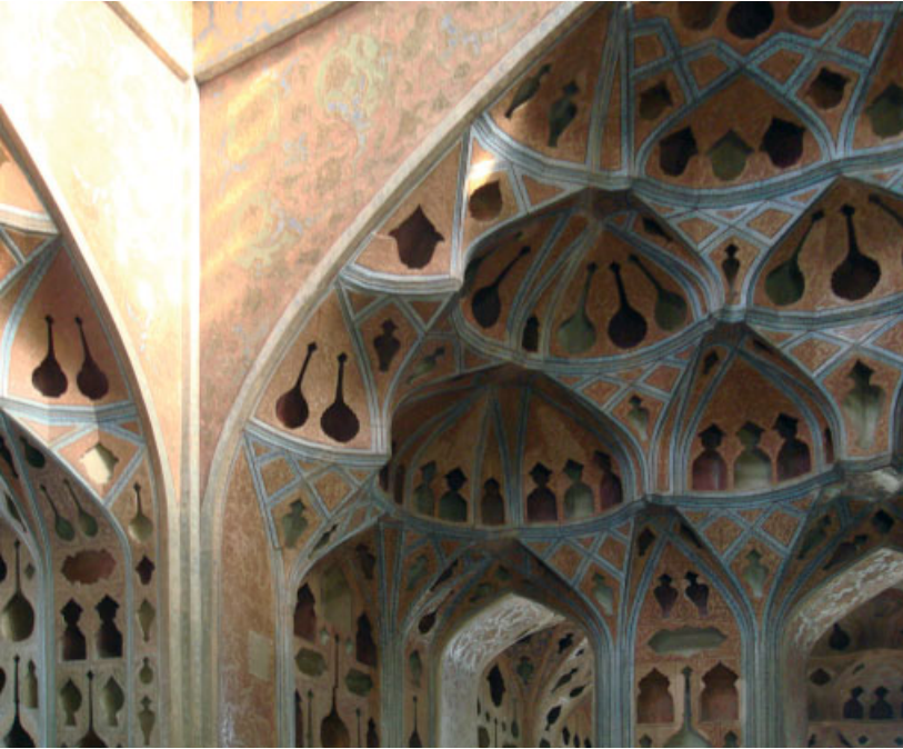
The walls and ceiling of the music chamber of the Ali Qapu palace in Isfahan, Iran, have cavities that are set into them with the purpose of reducing reverberation and holding upper and lower tones. In doing so they become an extension of the musical instruments, embedded within the architecture of the music chamber. The plasterwork is fantastically intricate, tapering to 3 millimetres (0.12 inches) thickness towards the edge of each cavity. Such work was possible due to an unprecedented accumulation of craftsmanship in one location.
