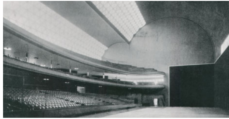
Eduardo Torroja, Fronton Recoletas stadium, Madrid, Spain, 1935 The roof of this pelota stadium is constructed as two asymmetrical cylindrical vaults. Although the appearance of the roof is largely that of a vault, the predominant structural action is that of a beam.
